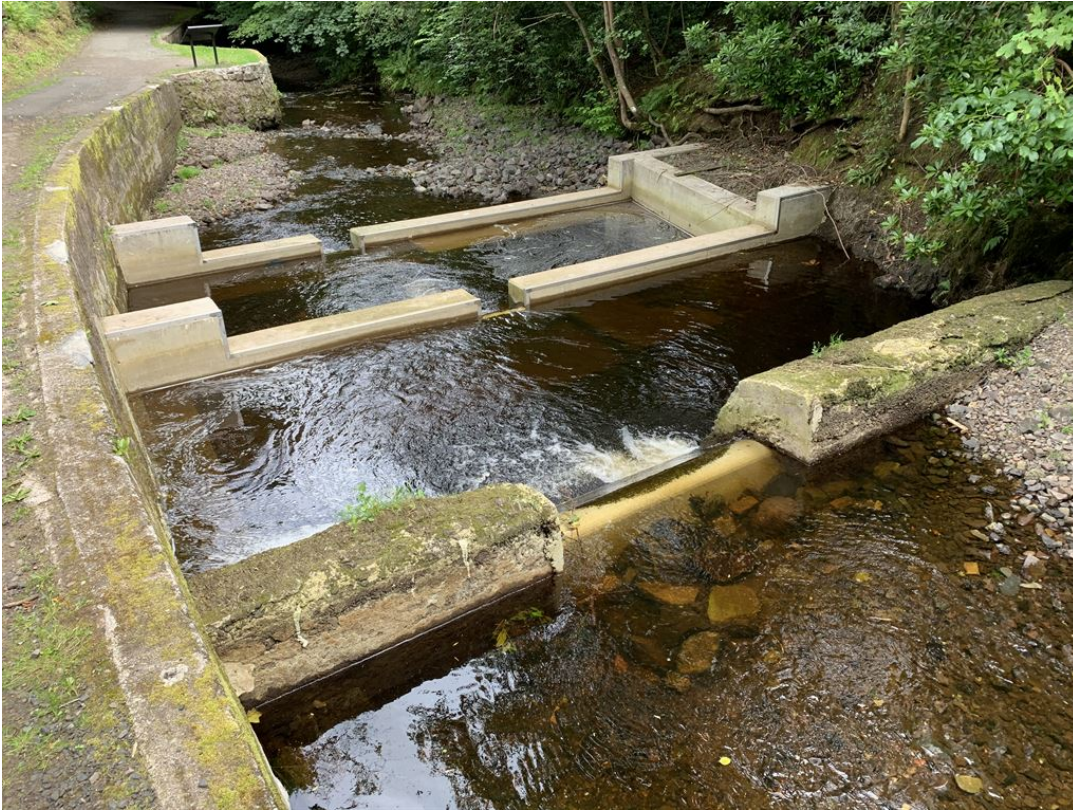
The water weir project at Gotter, Scotland
