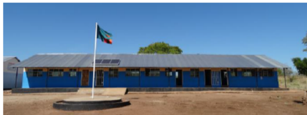
BrITE Foundation sponsored construction of toilet facilities in a new school building at Kasiya primary school in Zambia
