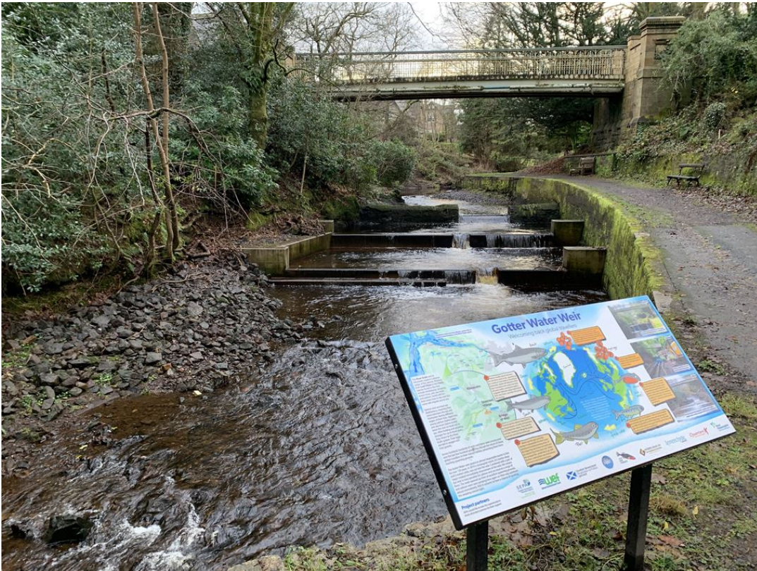
The water weir project at Gotter, Scotland
